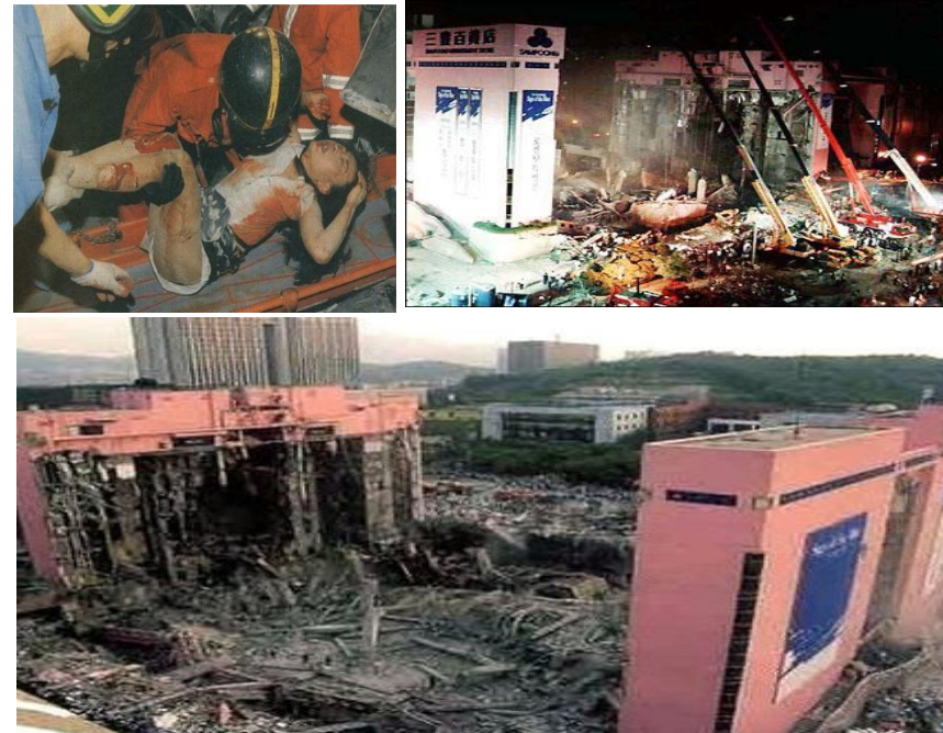
collapse of department store('95. 6) : 502 dead
