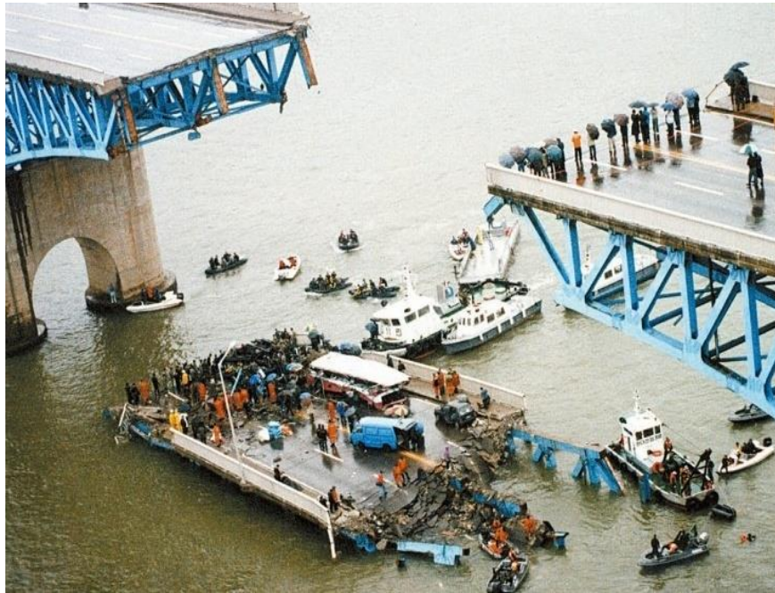
Bridge collapse ('94. 10) : 32 dead / 17 injured
