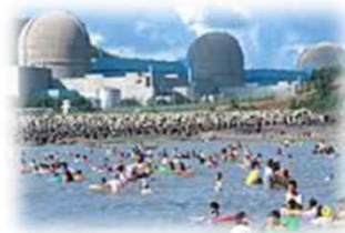
Nuclear Power Plant
