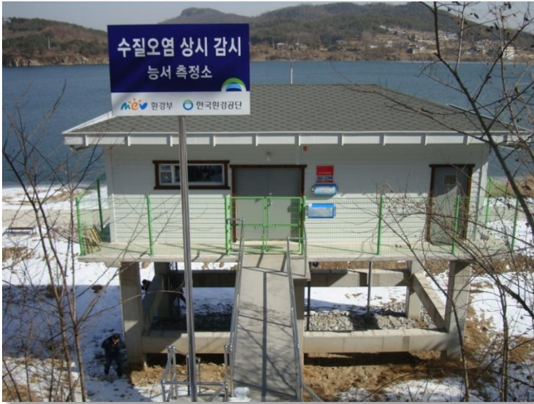
Outside vies of station building
