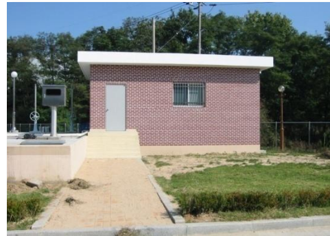
Outside views of station building
