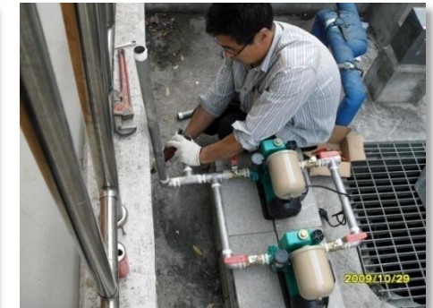
Sampling pump and pipe construction
