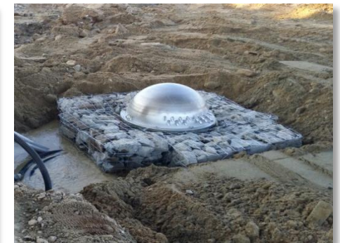
Sampling manhole installation
