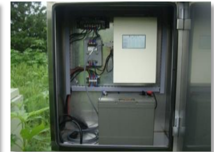
RTU installation
