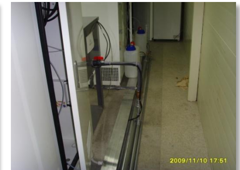
Pipe and electricity construction
