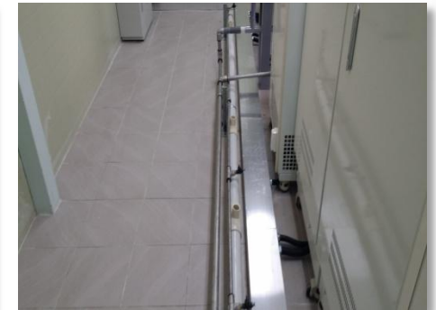
Pipe & duct installation
