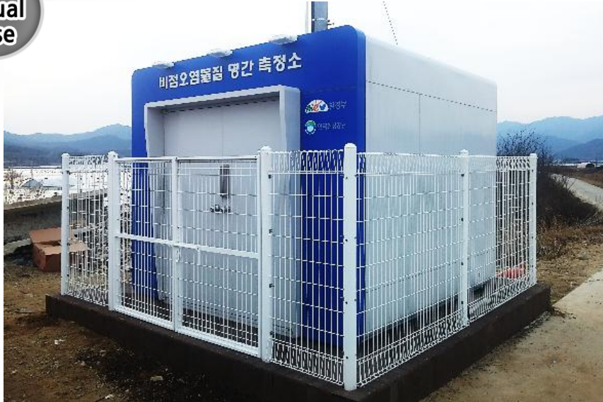
Outside vies of station building
