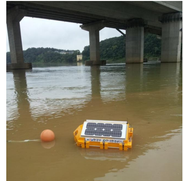
Mobile type monitoring system
