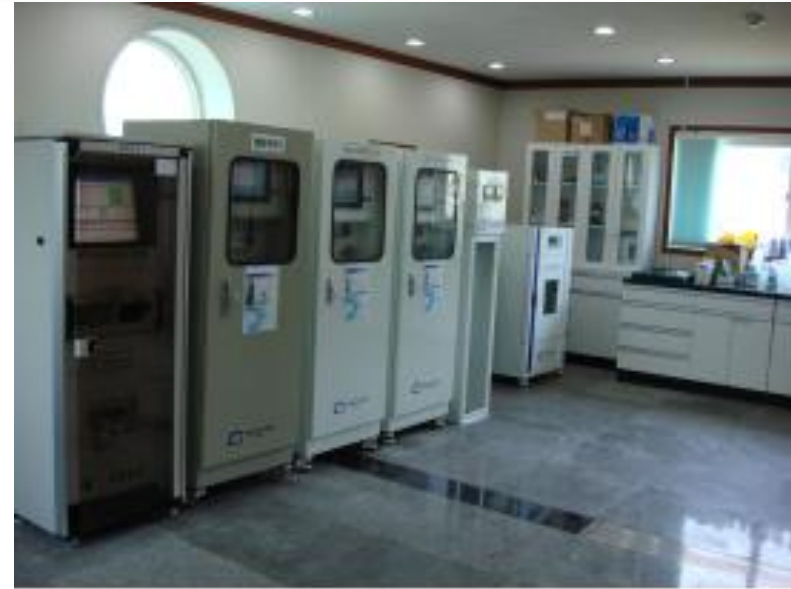
Inside view of station building
