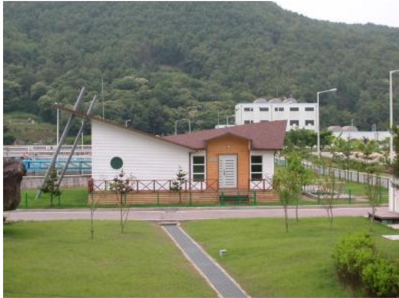
Outside vies of station building
