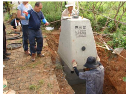
Concrete block reclamation
