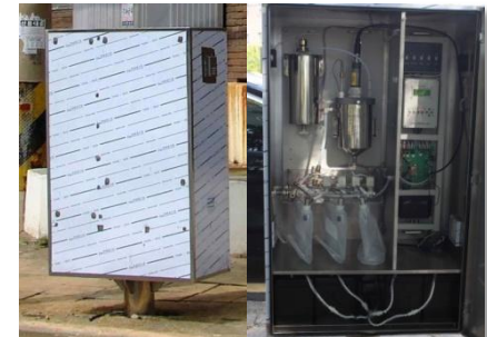
Controlboard and solar panel installation
