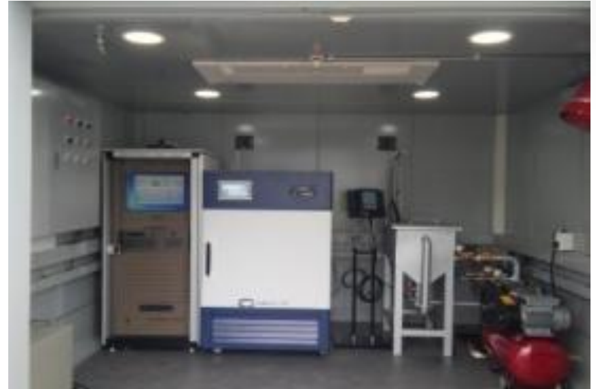
Inside station building
