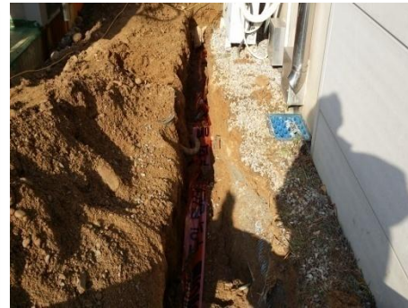
Sampling pipe construction
