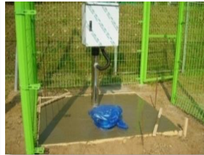
Support bean construction
