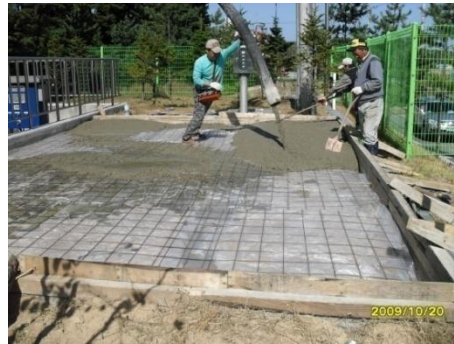
Concrete cast-in place
