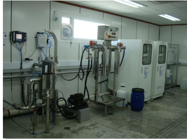
Inside view of station building
