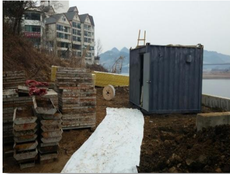
Construction site secure
