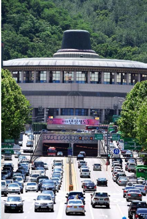
Woomyun Hill Tunnel
