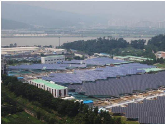
Amsa Arisu Water Purification Center(5MW)
