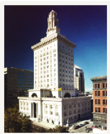
Seismic Retrofit: Oakland City Hall
