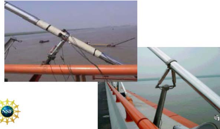
Wind Vibration Control of Stay-cables (Dong-ting Bridge, China)
