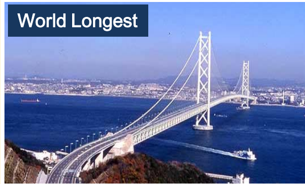
Akashi Bridge (1998), Japan Main Span - 1991m
