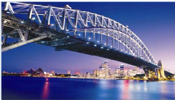
Bridge and Building Monitoring
