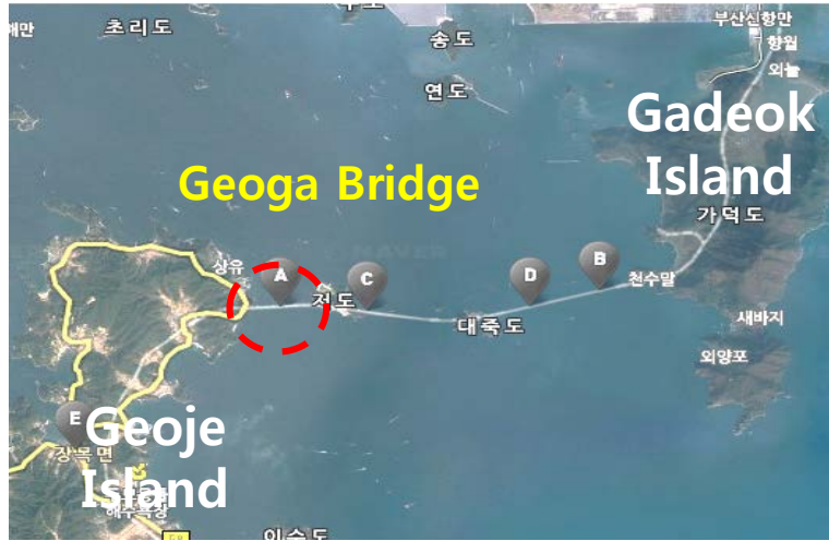
Geoga Cable-stayed Bridge
