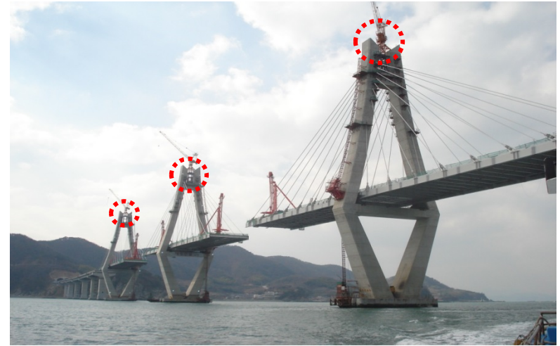
TMD Locations on Pylons
