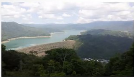
View of the dam
