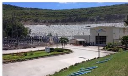
Power Plant House
