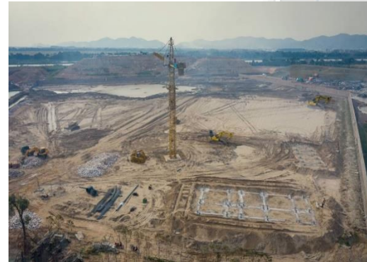
<Initial construction at the project site at the end of 2020>
