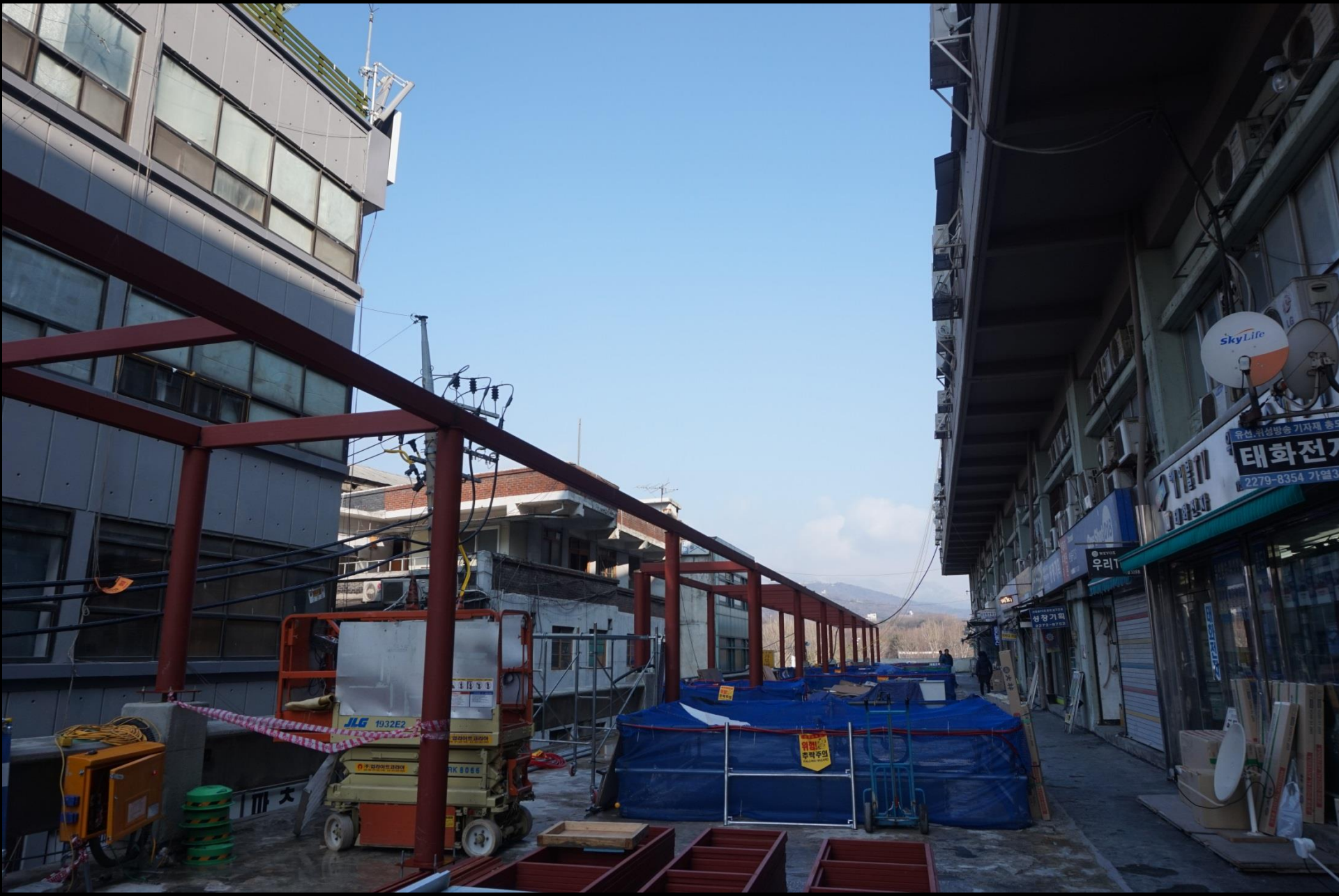
Maker's Cube at Sewoon Sanggu under Construction (Live Projects: Production City)
