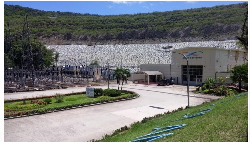
Power Plant House
