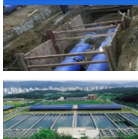
WTP / WWTP / Water Pipeline Construction
