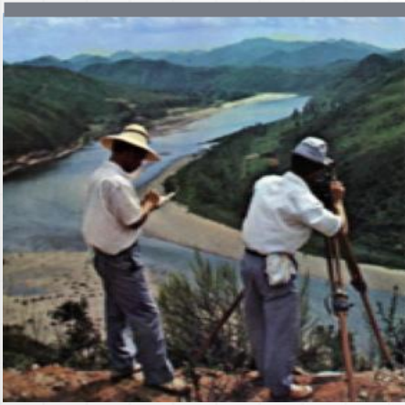
Investigation & Planning, First Dam Construction
